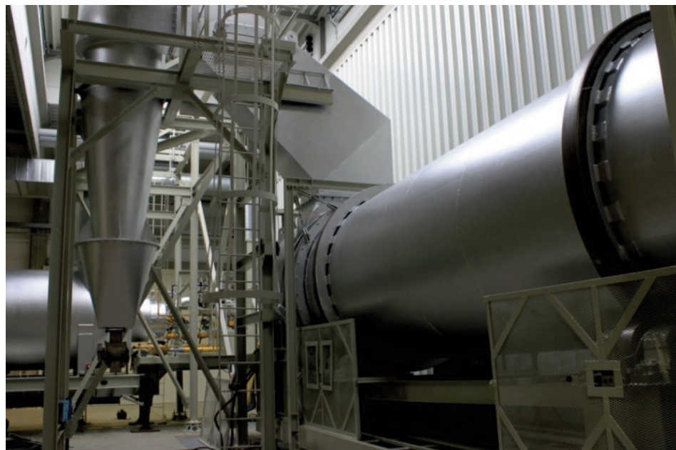
Figure 5-3: Rotary Kiln at the Remondis QR Site in Dorsten (Source: Remondis 2020)
